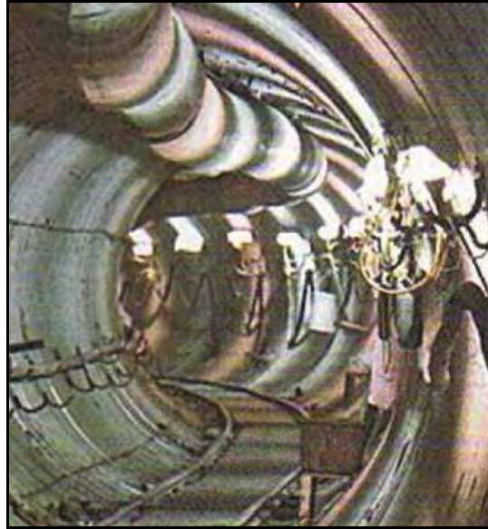
Figure 2-40: Tunnel Lined with Precast Reinforced Concrete Segments (Source: Yogi Kwong Engineers, Inc.)
