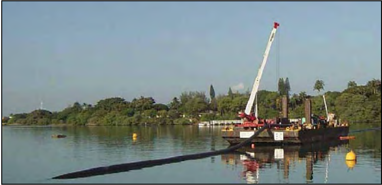
Figure 2-38: Over Water HDD Pipeline Pull Back (HPA Pipe) in Pearl Harbor
