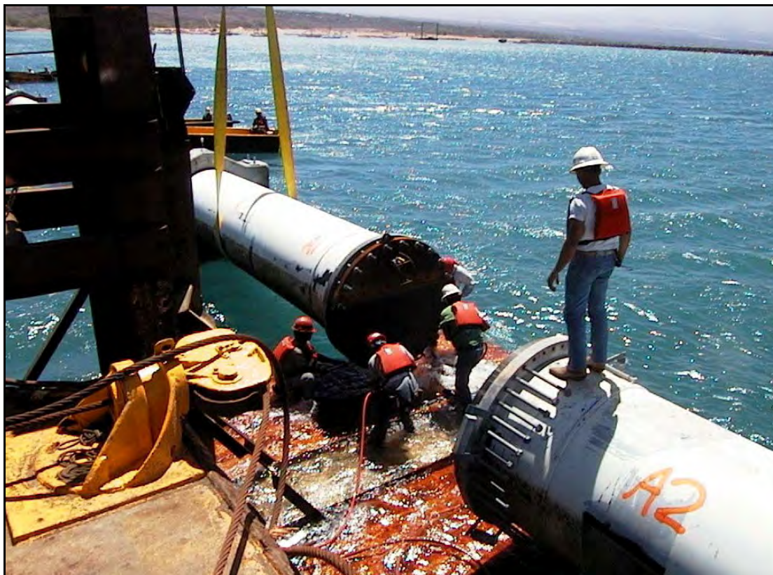
Figure 2-27: Assembling Flange Joints on Elevator Platform on Crane Barge (Source: Makai Ocean Engineering, Inc.)
