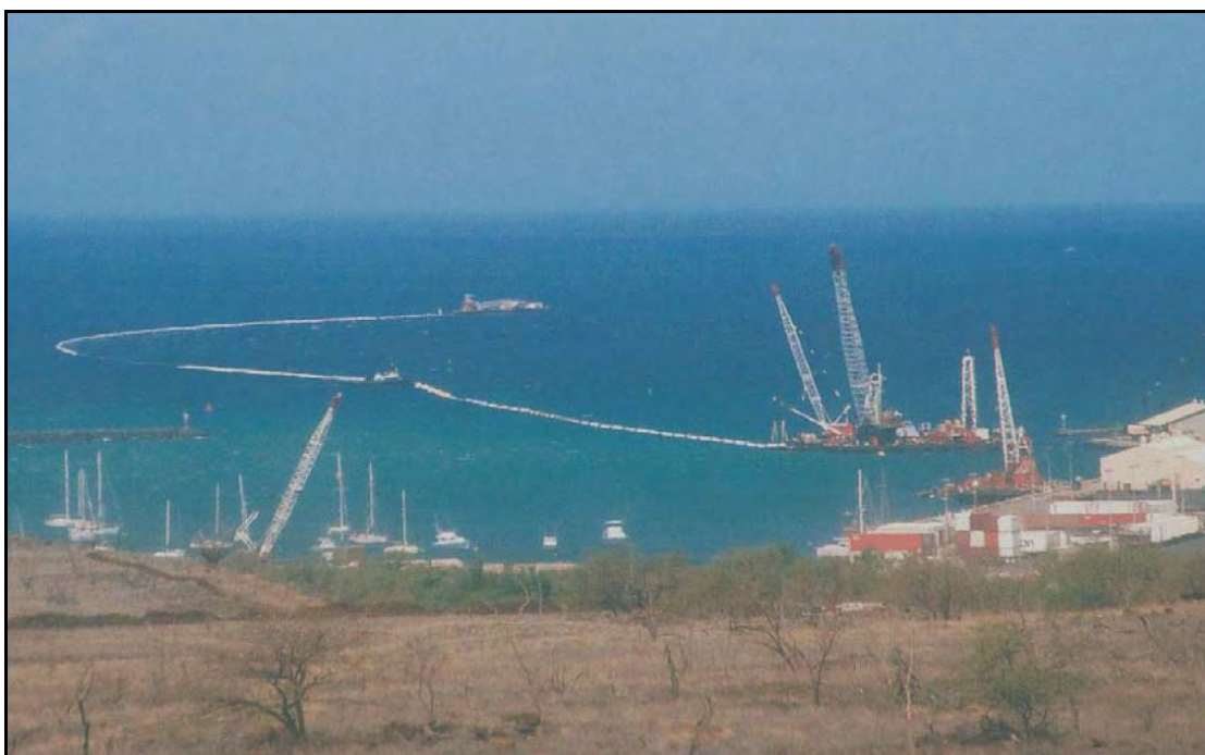
Figure 2-28: Fully Assembled NELHA 55-inch Pipe Being Towed From Kawaihae Harbor (Source: Makai Ocean Engineering, Inc.)
