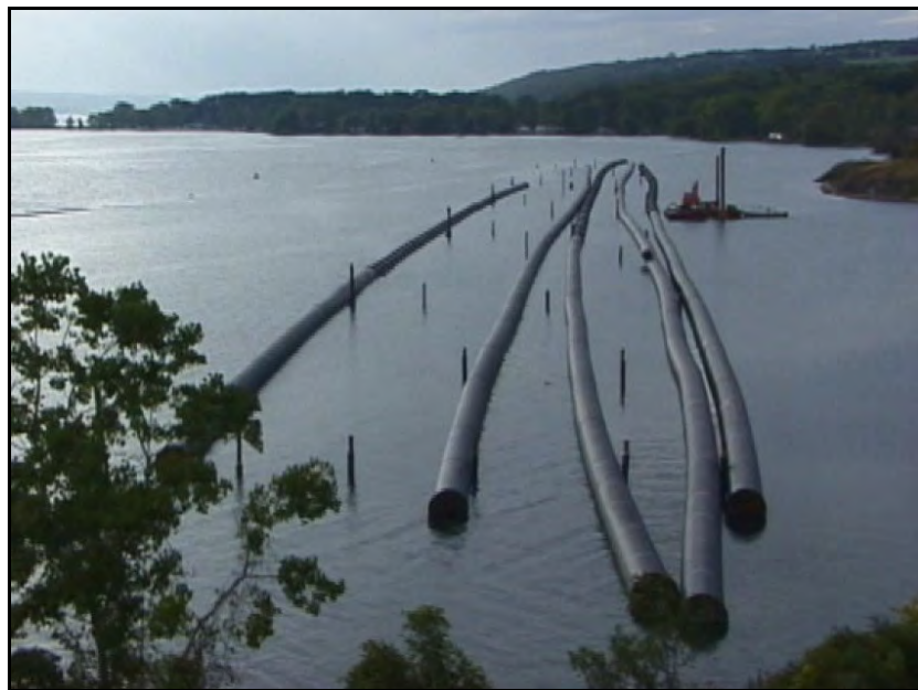
Figure 2-25: Stored Floating Pipeline with Stiffeners and Anchor Weights Being Attached
