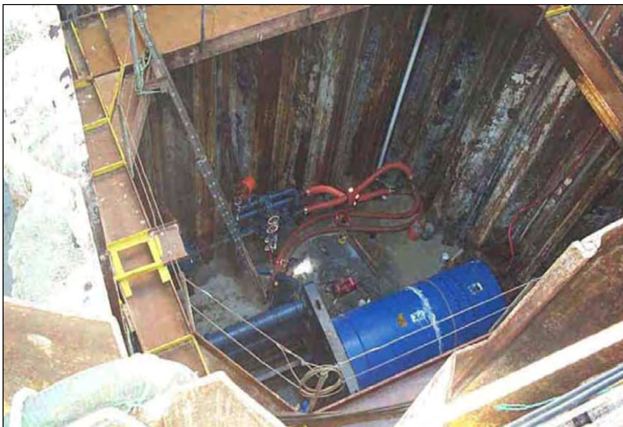
Figure 2-6: Forty-foot Deep Microtunnel Pit off Pearl Harbor (Source: Yogi Kwong Engineers, Inc.)
