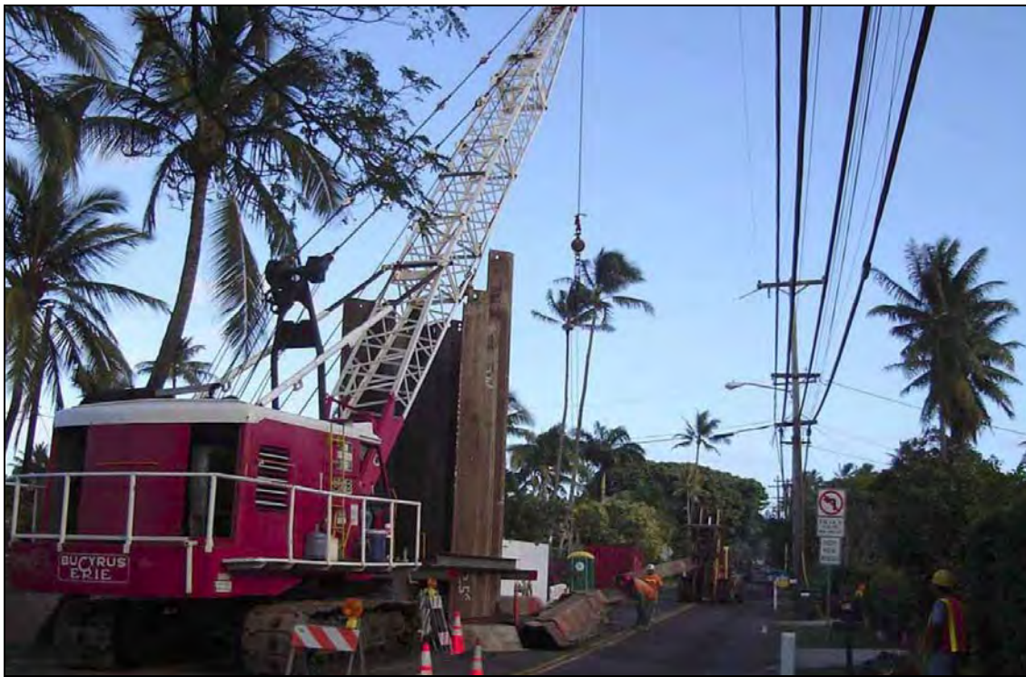
Figure 2-4: Microtunnel Jacking Pit Construction on a Narrow Public Roadway in Kailua, O'ahu (Source: Yogi Kwong Engineers, Inc.)
