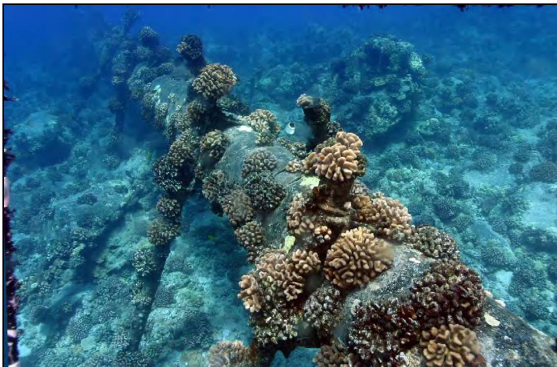
Figure 3-33: Photo of an HDPE Coldwater Pipeline at the Natural Energy Laboratory of Hawaii at Keāhole Point, Hawai'i, Showing Coral Development
