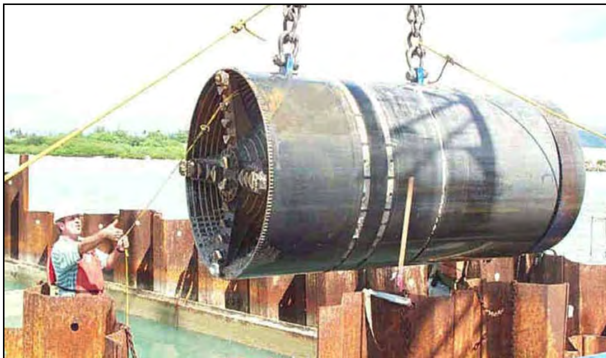
Figure 2-7: Wet Retrieval of Microtunnel Boring Machine (Source: Yogi Kwong Engineers, Inc.)
