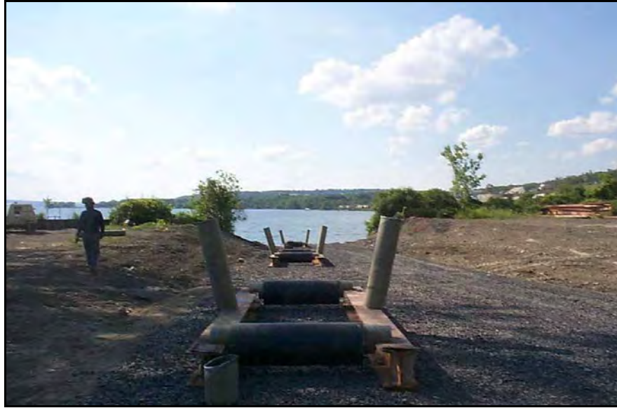
Figure 2-24: Roller Bed to Launch HDPE Pipe into Water
