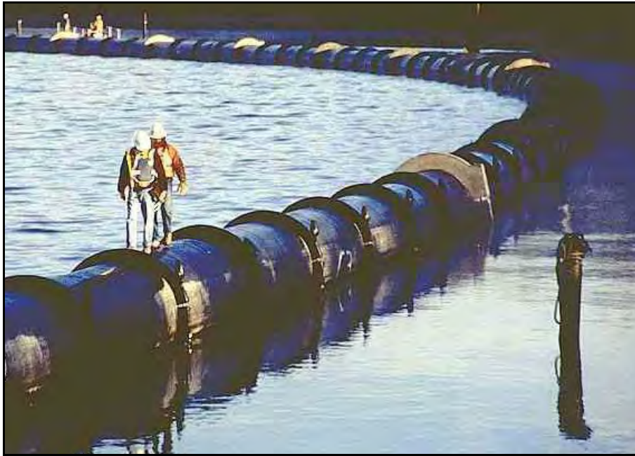
Figure 2-16: A 63-inch Pipeline with Ductile Iron Stiffeners and Anchor Collars (Source: Makai Ocean Engineering, 2005a)
