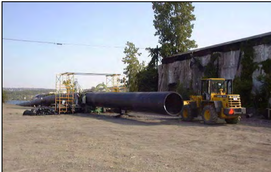
Figure 2-23: HDPE Pipe Fusion Operation (Source: Makai Ocean Engineering, Inc.)
