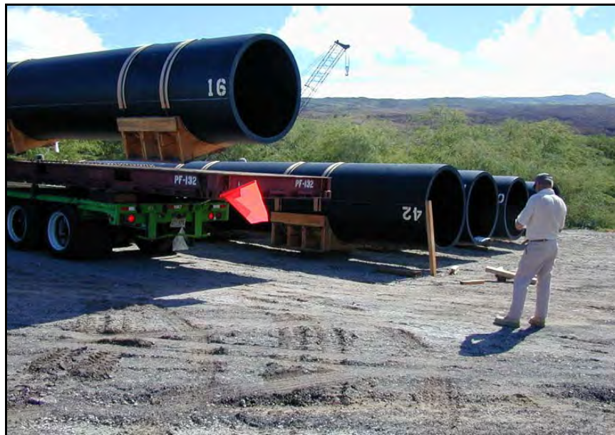
Figure 2-21: Large Diameter HDPE Pipe Being Unloaded and Stored at Kawaihae Harbor (Source: Makai Ocean Engineering, Inc.)
